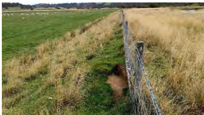
Figure 3.4 Low risk of embankment breach. Slumping of the embankment crest appears to have been caused by livestock trampling. The embankment is set back from the riverbank and signs of slumping observed are localised.
