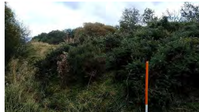
Figure 3.9. Scrub growth on the crest and face of an embankment.
