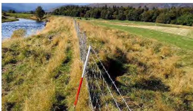
Figure 3.5 Moderate risk of embankment breach. Situated within 5 m of the riverbank, with slumping and bare ground exposed on the dry side of the embankment.
