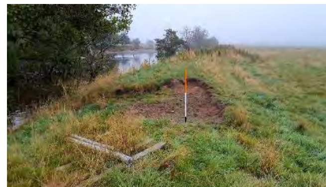
Figure 3.6 High risk of embankment breach. Embankment positioned along the top of the riverbank. Bare ground and slumping evident across over half of the embankment crest width.
