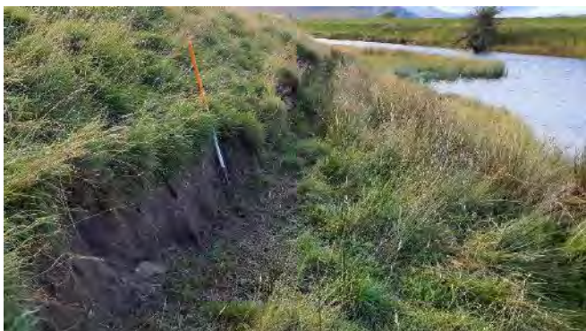
Figure 3.1. Low-severity riverbank erosion.
