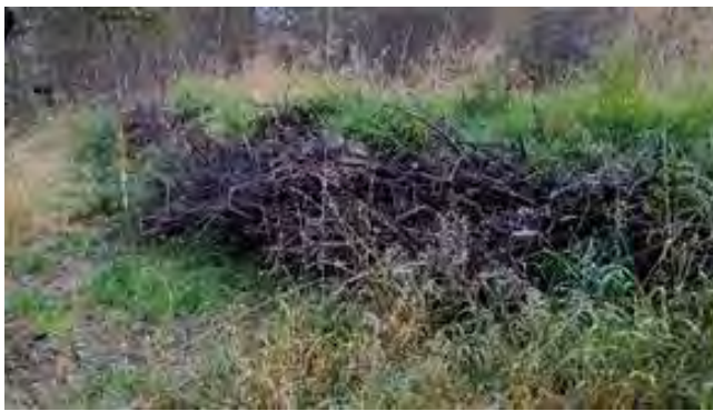
Figure 3.61 Example embankment breach remedial works. Large wood (trunks with root plates still attached) installed to protect the embankment face (OS NGR NH 88320 09028).
