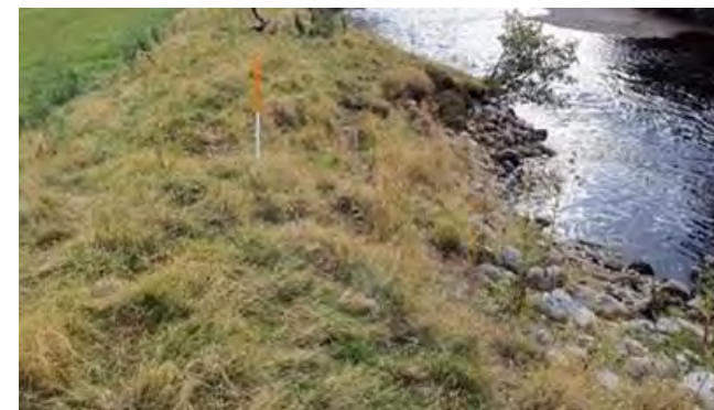
Figure 3.12 Riverbank erosion undermining an embankment positioned at the top of the bank. High risk of embankment breach.
