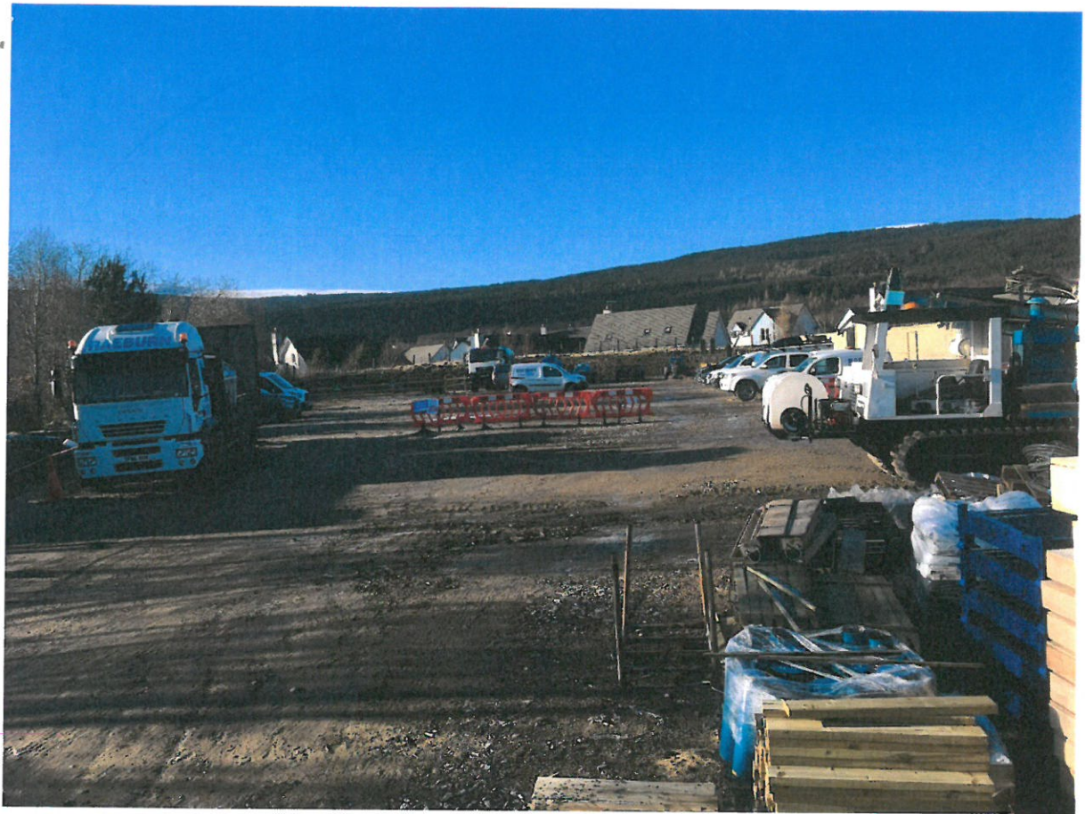
The site looking from the entrance
