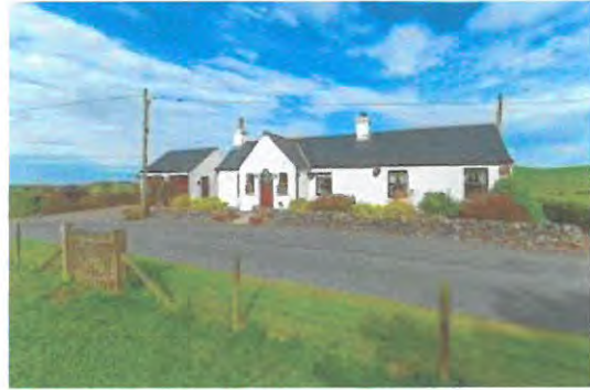
Vernacular Highland Cottage
