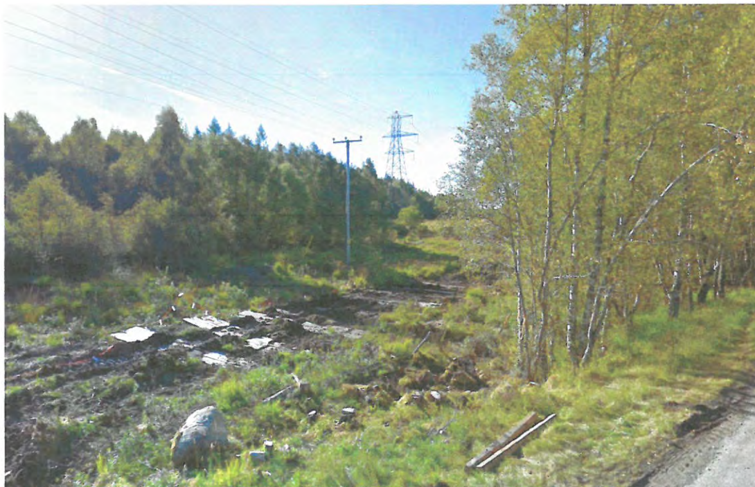
Site showing National Electricity Distribution Pylon
