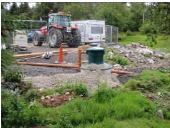
**Fig. 4: Newly developed septic tank**
