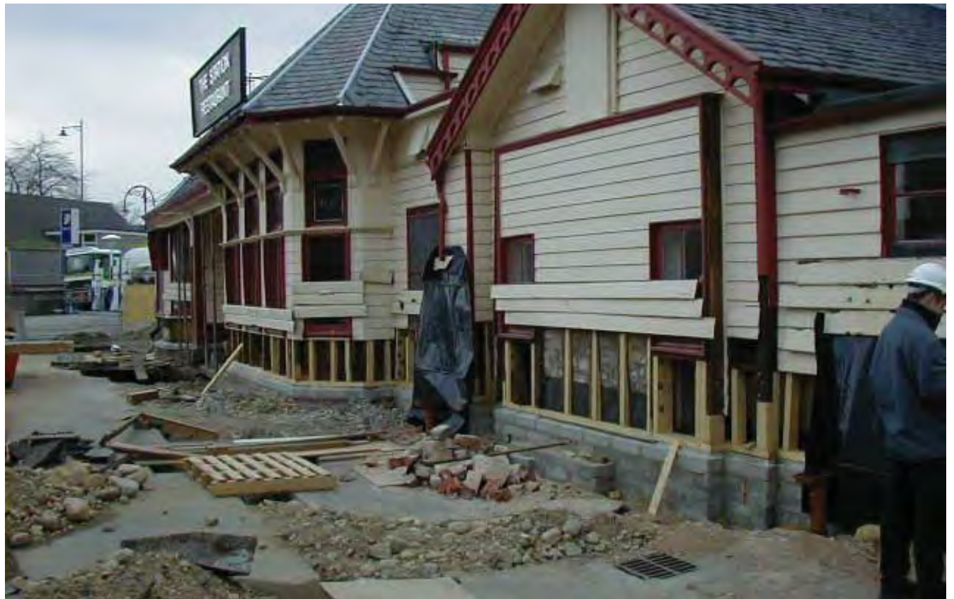
Underbuilding work being carried out.
