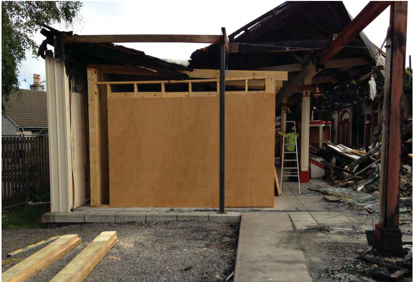
Erection of Royal Carriage enclosure
