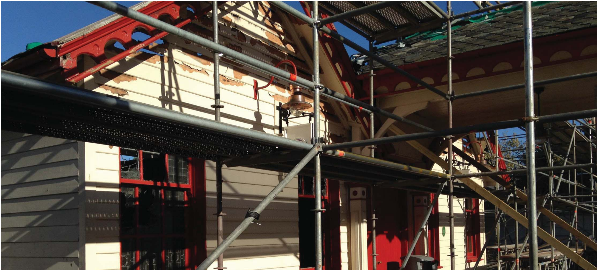
Erection of Temporary Enclosure
