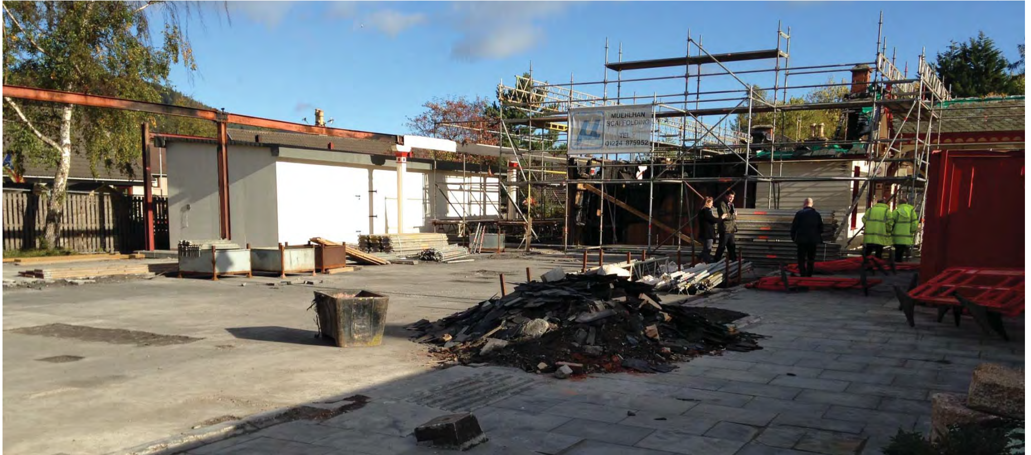
Erection of Temporary Enclosure
